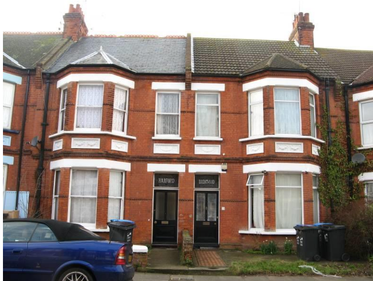
Houses like these in Warwick Road would be protected from unsympathetic alterations by an Article 4 Direction
