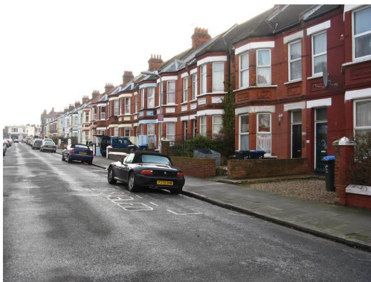
Warwick Road – west side
