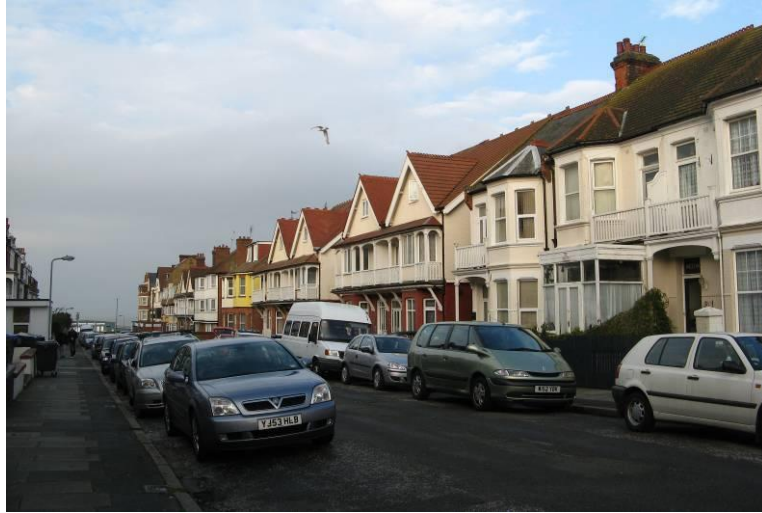
These properties in Surrey Road were mainly built in the 1920s
